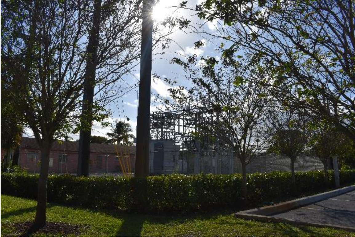
View looking southwesterly from adjoining commercial use
