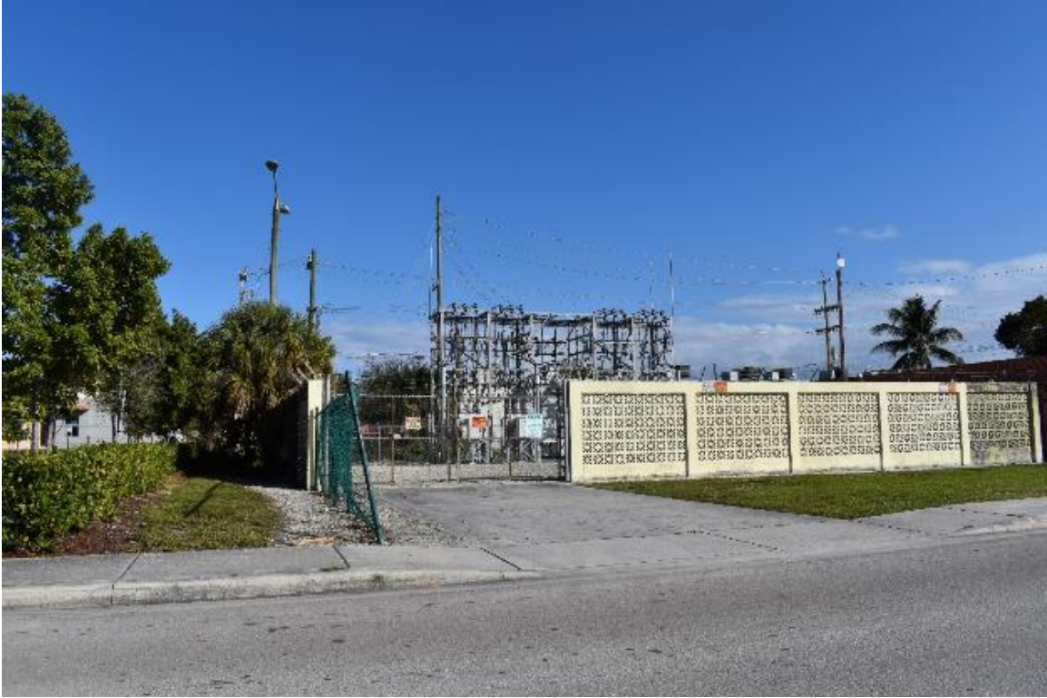
View looking easterly of driveway on South H Street
