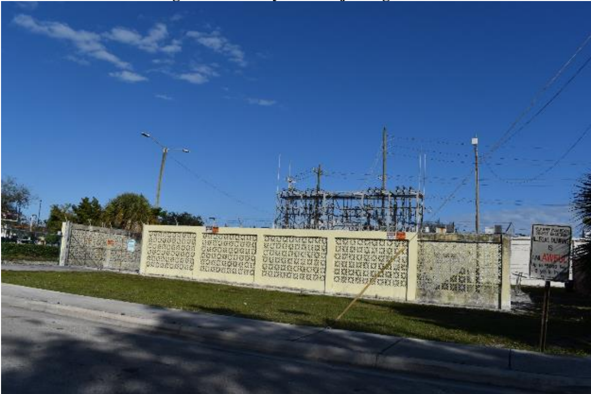
View looking northeasterly of South H Street frontage
